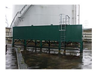
The power station at Kings Lynn needed to preserve a 50,000-liter fuel storage tank that was not being used and was unlikely to be used in the near future. The power station staff was concerned that the tank could start to corrode, particularly from the inside out, due to the fact that the inside of the tank was bare metal. According to Cortec, its VpCI®-705 was chosen to protect the tank because:
