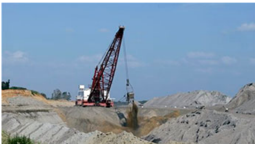
In this July 29, 2013, photo, a Dragline excavator works a strip mine near Tatum, Texas. Decades of mining and power plant activity that helped East Texas towns grow and thrive could be threatened as a large energy provider faces possible bankruptcy. (AP Photo/LM Otero)
