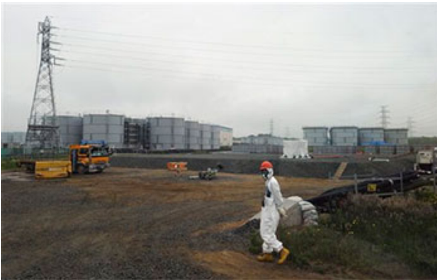
In this Wednesday, June 12, 2013 file photo, a construction worker walks beside the underground water tanks at the Fukushima Dai-ichi nuclear plant at Okuma in Fukushima prefecture, Japan. The operator of Japan's tsunami-crippled nuclear power plant said Tuesday, Aug. 20, 2013, that about 300 tons of highly radioactive water have leaked from one of the hundreds of storage tanks there - its worst leak yet from one of the vessels. (AP Photo/Toshifumi Kitamura, Pool)
