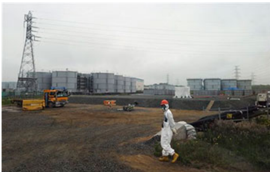
In this Wednesday, June 12, 2013 file photo, a construction worker walks beside the underground water tanks at the Fukushima Dai-ichi nuclear plant at Okuma in Fukushima prefecture, Japan. The operator of Japan's tsunami-crippled nuclear power plant said Tuesday, Aug. 20, 2013, that about 300 tons of highly radioactive water have leaked from one of the hundreds of storage tanks there - its worst leak yet from one of the vessels. (AP Photo/Toshifumi Kitamura, Pool)
