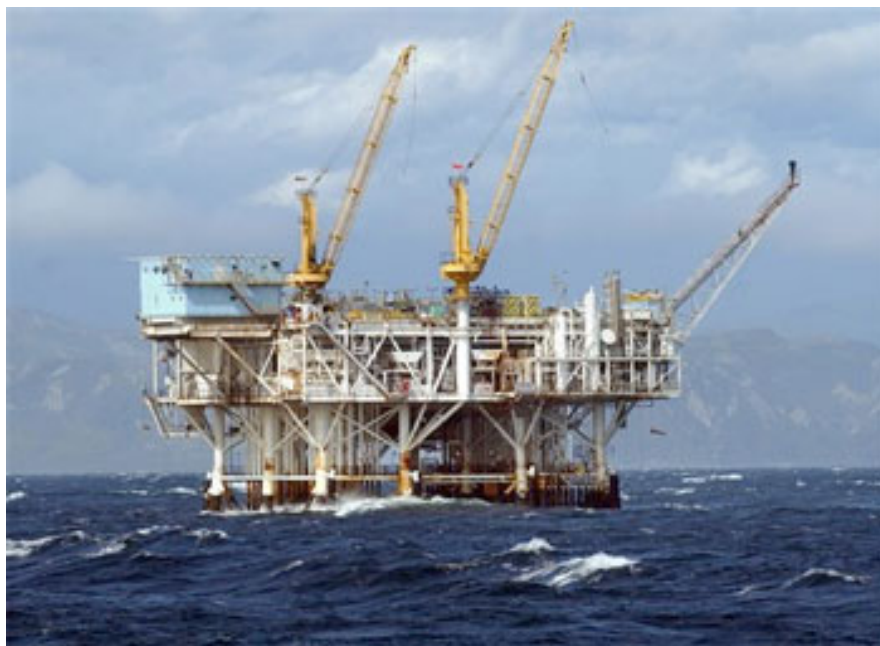
This file photo taken April 12, 2005 shows the oil platform Gilda is seen in federal waters in the Santa Barbara Channel off Ventura, Calif. Several California lawmakers have sent a letter to the federal government asking for an investigation into hydraulic fracturing, or fracking, off the California coast. (AP Photo/The Santa Barbara News-Press, Steve Malone, file)
