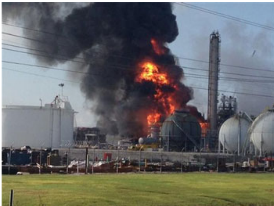
This photo provided by Ryan Meador shows an explosion at The Williams Companies Inc. plant in the Ascension Parish town of Geismar La., Thursday, June 13, 2013. The fire broke out Thursday morning at the plant, which the company's website says puts out about 1.3 billion pounds of ethylene and 90 million pounds of polymer grade propylene a year. (AP Photo/Ryan Meador)
