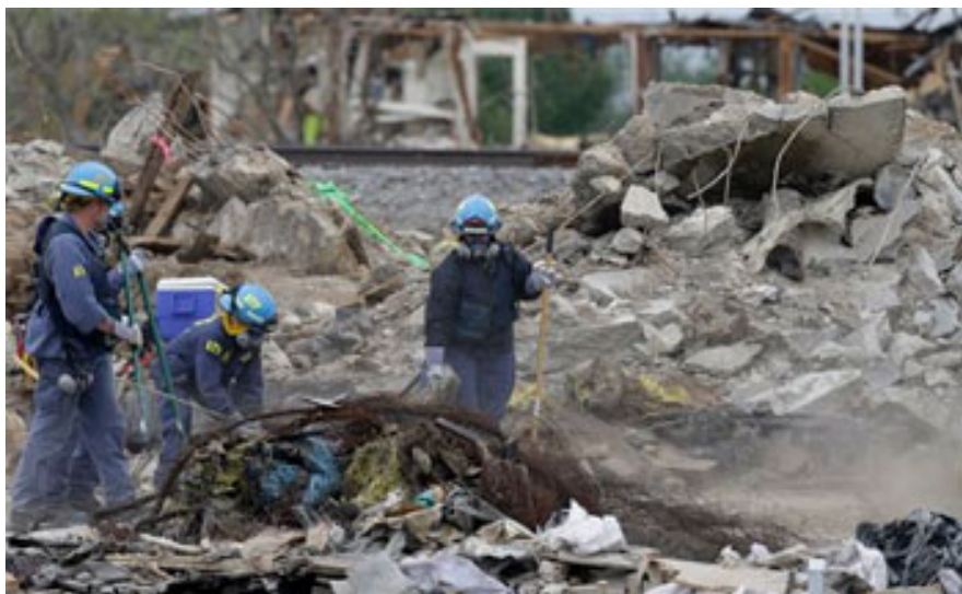
Investigators sift through the debris of the destroyed fertilizer plant in West, Texas, Thursday, May 2, 2013. Investigators face a slew of challenges in figuring out what caused the explosion at the fertilizer plant that killed 14 people and destroyed part of the small Texas town. (AP Photo/LM Otero, Pool)
