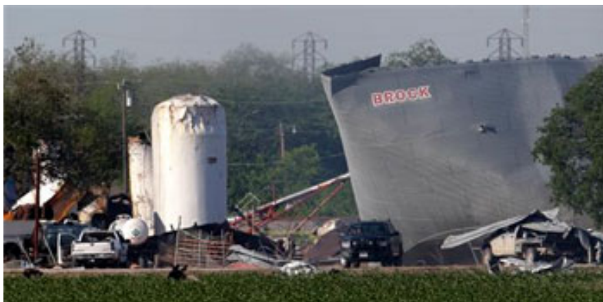
Law enforcement personnel patrol the scene Saturday, April 20, 2013, three days after an explosion at a fertilizer plant in West, Texas. The massive explosion at the West Fertilizer Co. Wednesday night killed at least 14 people and injured more than 160. (AP Photo/Charlie Riedel)
