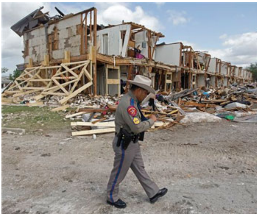
Texas Department of Public Safety Sgt. Jason Reyes walks past a damaged apartment complex, Sunday, April 21, 2013, four days after an explosion at a fertilizer plant in West, Texas. The massive explosion at the West Fertilizer Co. Wednesday night killed 14 people and injured more than 160. (AP Photo/The Dallas Morning News, Michael Ainsworth, Pool)
