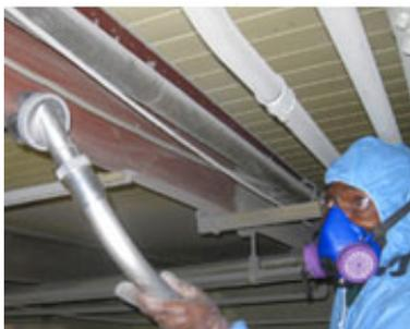
*This technician cleans combustible dust with explosion-proof vacuum equipment.*
