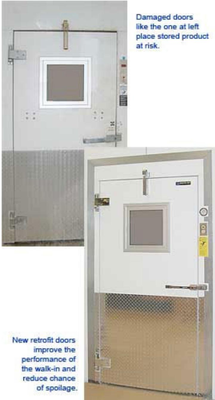
Food and beverage manufacturers rely on walk-in coolers and freezers for safe and efficient storage of perishable fresh and frozen food. Over the years, they have evolved to satisfy many needs of the food manufacturing industry from warehousing ingredients to serving as temperature control and holding stations for ready-to-ship product. As the uses for walk-in coolers have grown, so has their design and technology.
