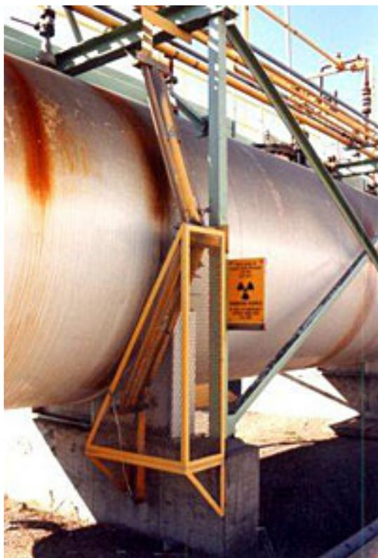
*Here's a close-up of nuclear rod sources mounted on a horizontal tank.*
