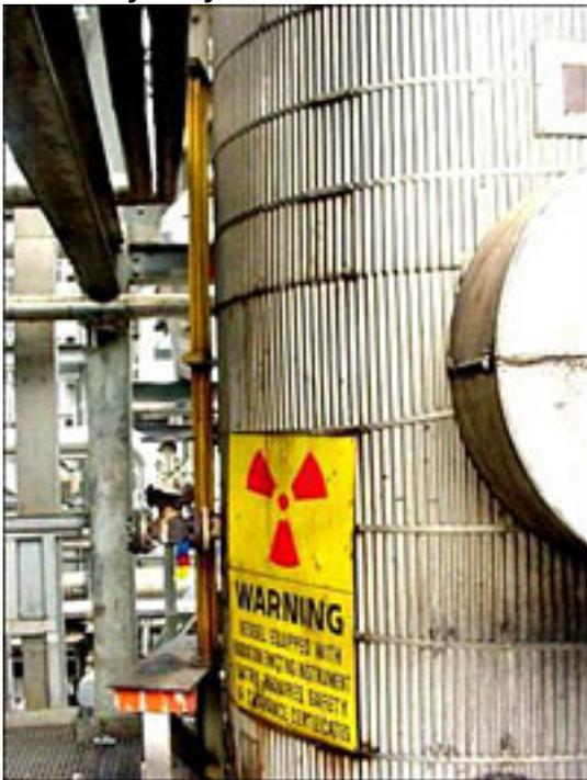
*A rod-type nuclear source is mounted on the outside of a vessel.*
